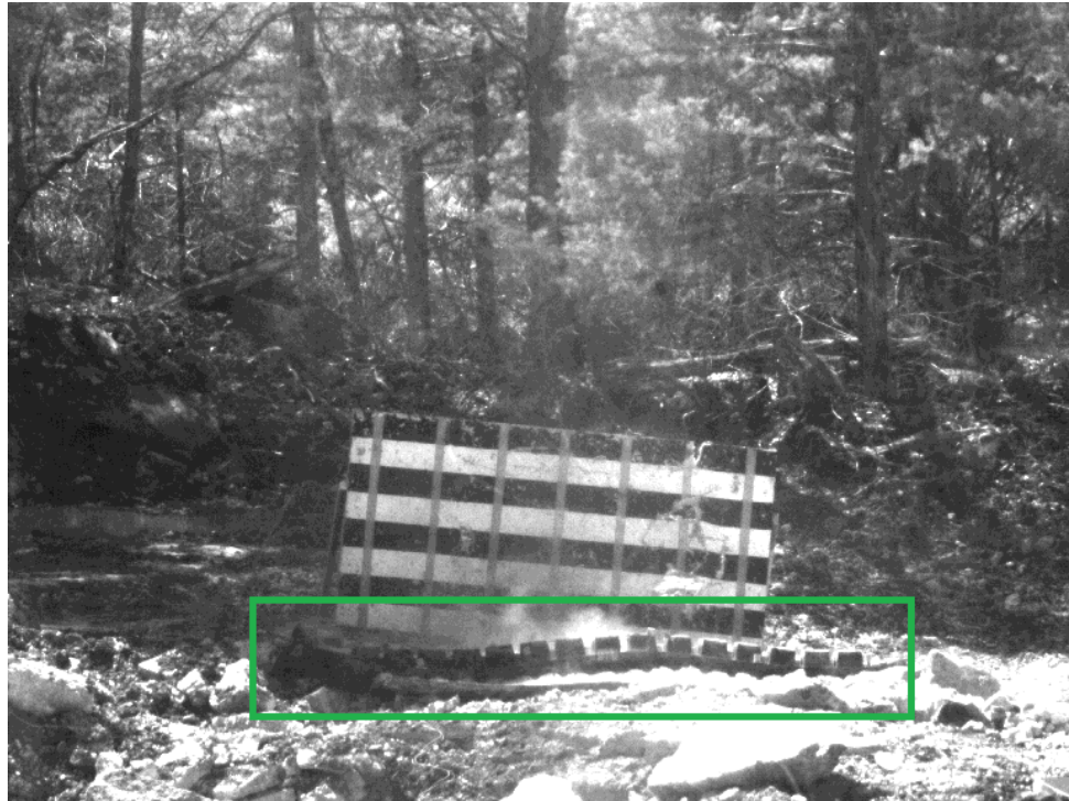
Figure 6.1 Blasting Mat Centered Over Borehole
